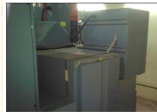
Right side view of right most bus bar VT - Thermal anomaly
