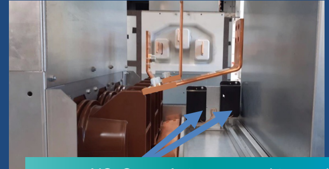
AIS: Same Antennas used to receive temperature values from SAW sensors will be used for partial discharge detection
