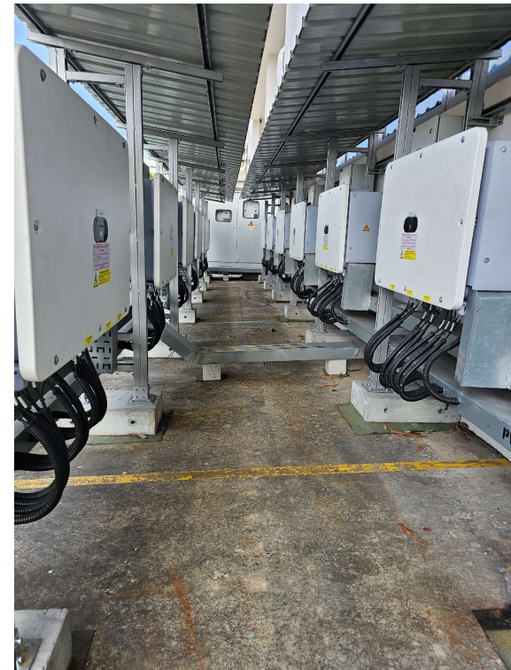
Now (3P 115kW transformerless inverter)
