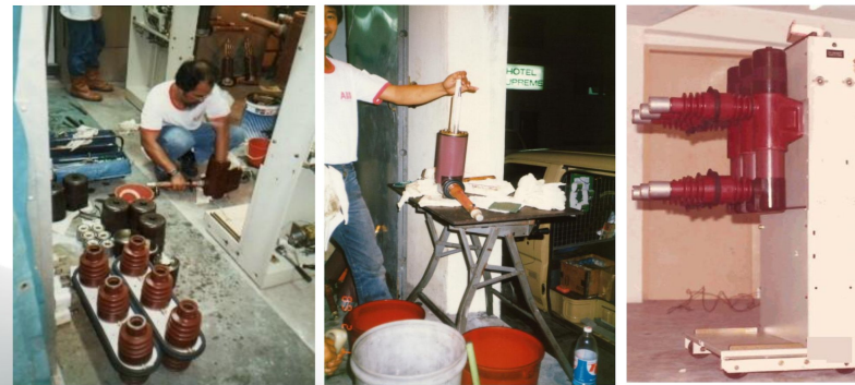
Complete overhaul of circuit breaker
