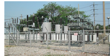
115 kV C-Bank, PEA For utility grids
