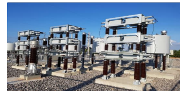
115 kV C-Bank, EDC For utility grids
